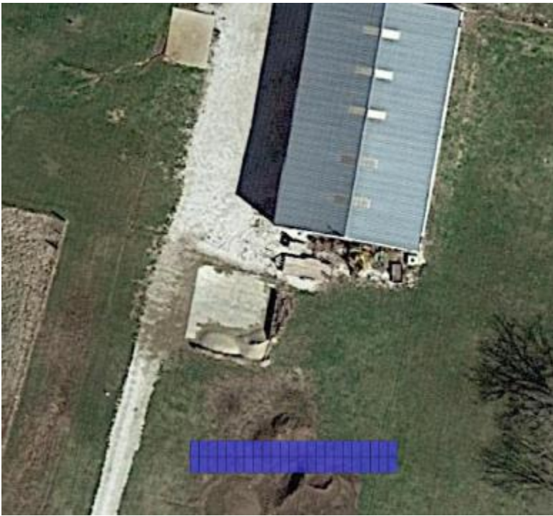
Maintenance: 4092 Hwy JJ
